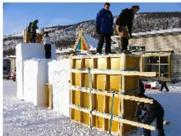
5. Building the tail.
