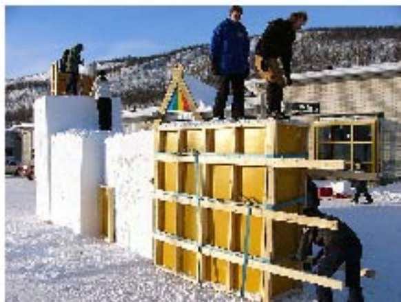
5. Building the tail.
