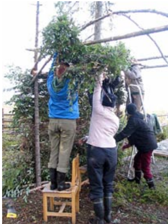
4. Collaboration in covering the roof
