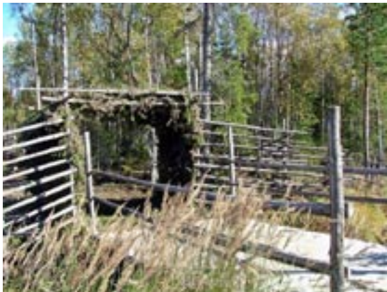
1. Old gate was a wood construction
