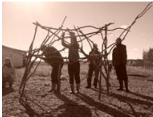
4. Building the framework of the cow Photo: Liisa Kotila
