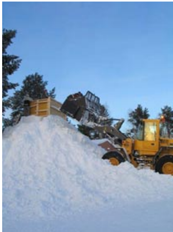
5. Construction of the ski jump
